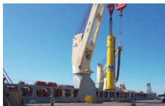
Installation of 72 monopiles on Kriegers Flak windfarm in record time
