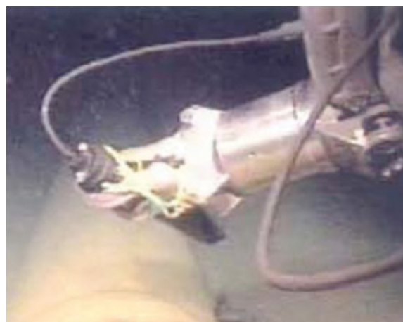
Standard cathodic protection A subsea photo of a standard cathodic protection survey (T-Handle not in use)
