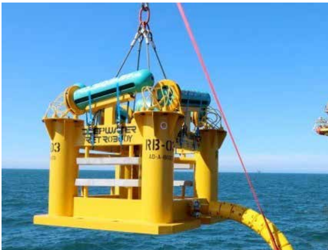
Photo: Deepwater's RetroBuoy remote anode sled being over-boarded
