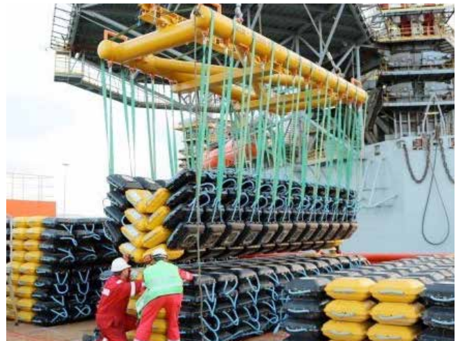
Photo: FLXMAT System concrete mattresses and 'Fast Lift' frame
