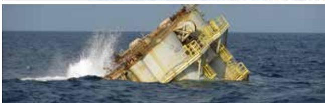
Photo: Vessels - B50 (ballasting, towing, reefing and mooring disconnect) and Kirt Chouest (mooring line-disconnect and recovery)
