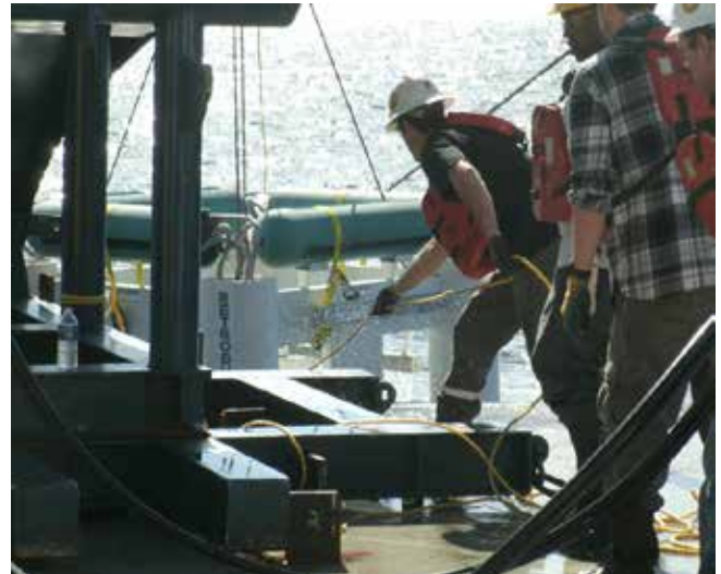
Photo: After each Retrobuoy is terminated and installed on the sea floor, it is hooked up to a transformer rectifier on the platform deck.
