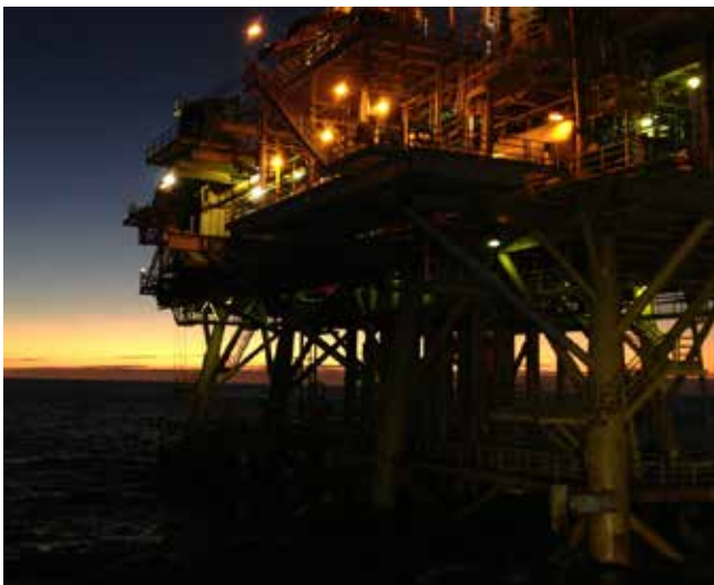
Photo: EW-305-A This platform is situated in the Gulf of Mexico in 300 ft of seawater.
