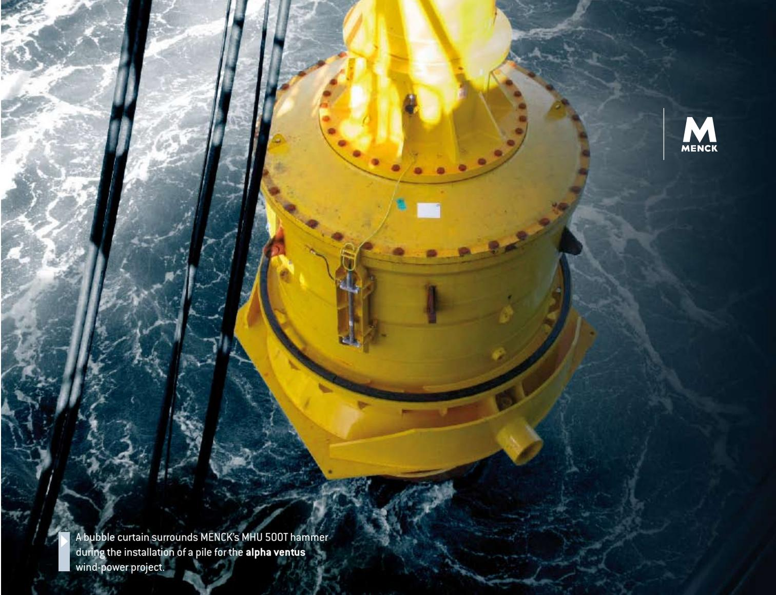
▶ A bubble curtain surrounds MENCK's MHU 500T hammer during the installation of a pile for the **alpha ventus** wind-power project.
